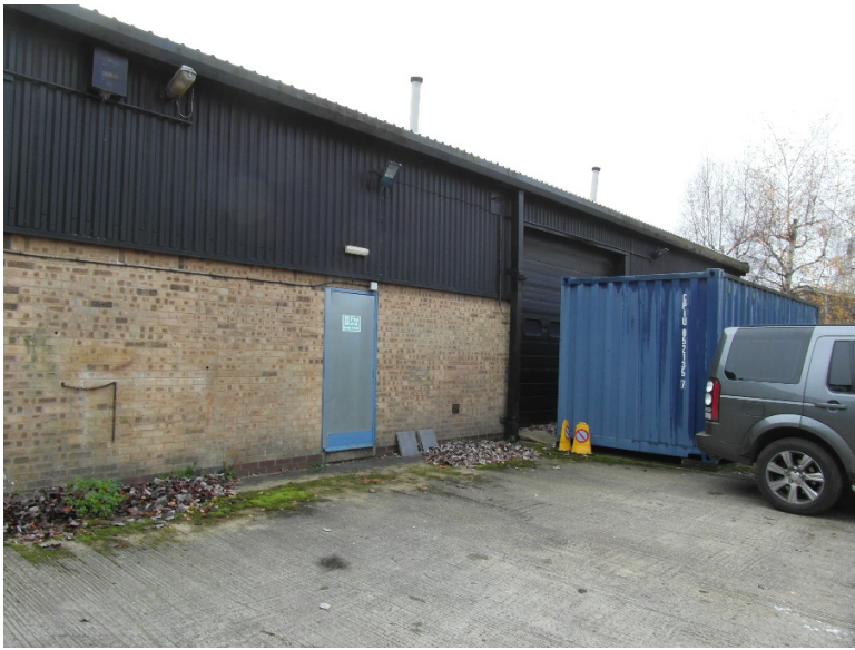
Rear fire exit from Lodge room
