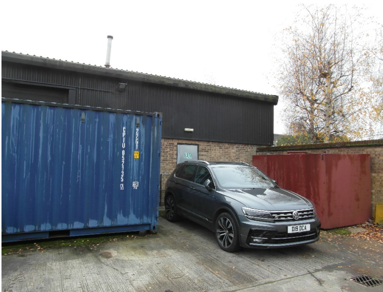
Rear fire exit from main hall
